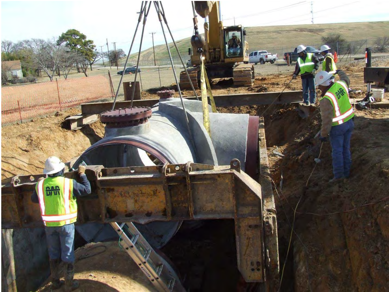
Picture 4 – Lowering tee into place on Kennedale Line J Section 1C
