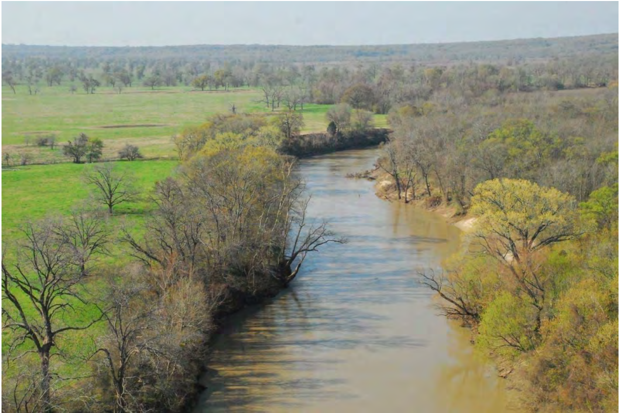
Figure 2-5. Trinity River Crossing (Facing South)
