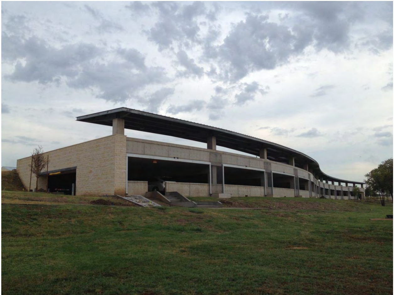
Picture 8 - Administration Parking Garage
