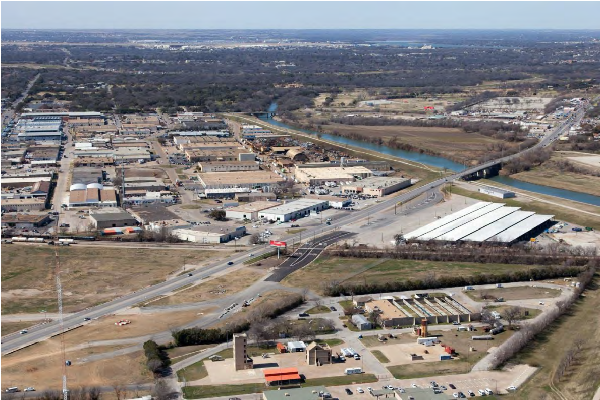
Picture 5 – New blacktop laid to detour Henderson St. traffic during construction
