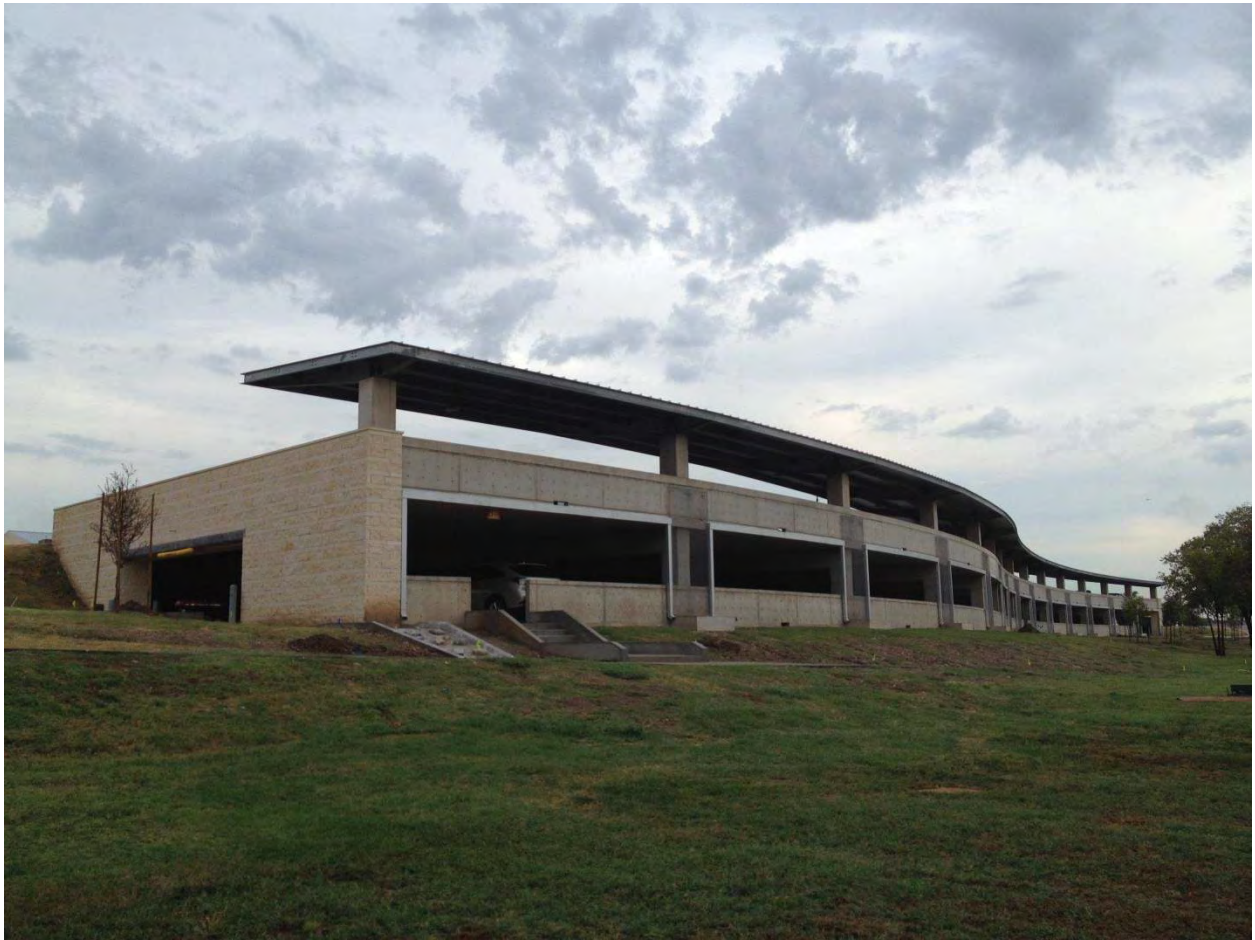
Picture 8 - Administration Parking Garage
