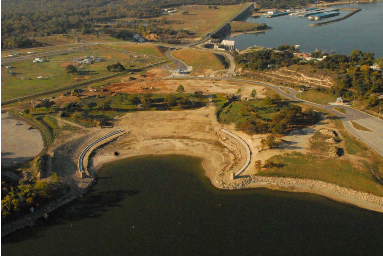
Picture 9 – Twin Points Park Swim Beach Retaining Walls
