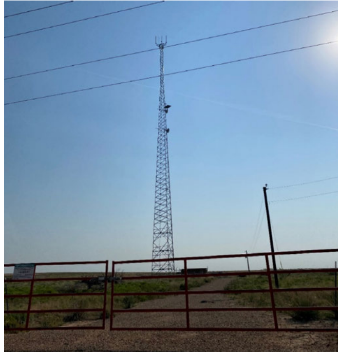
Figure 9 – FCC Free-Standing Communication Tower
