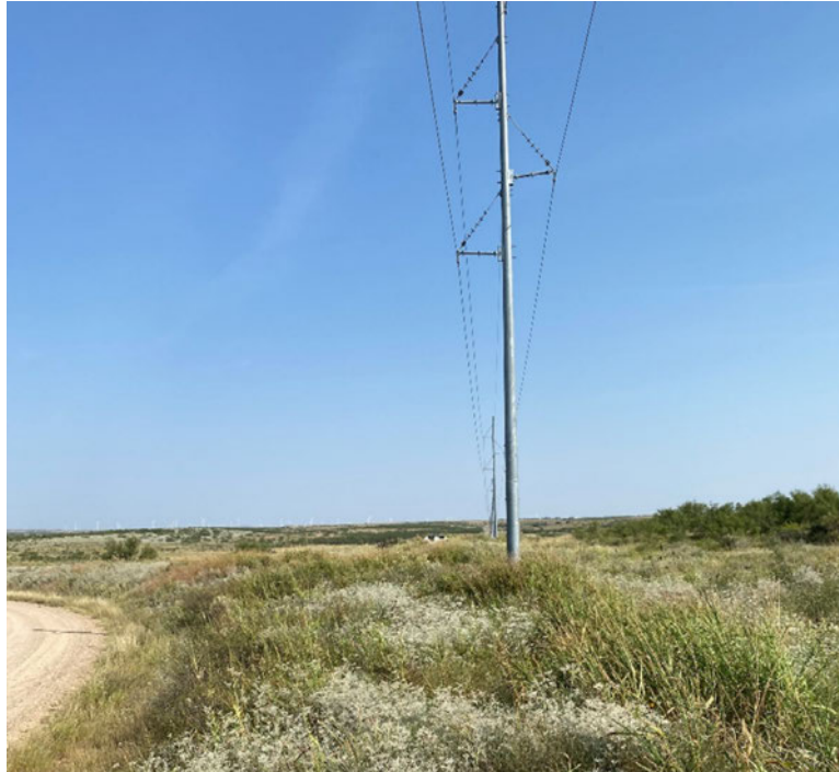
Figure 14 – Existing Electric Transmission Easement Along County Road I, Facing North
