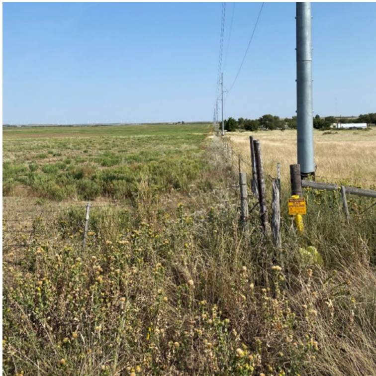
Figure 16 – Photo Taken Along Hereford Drive, Facing North
