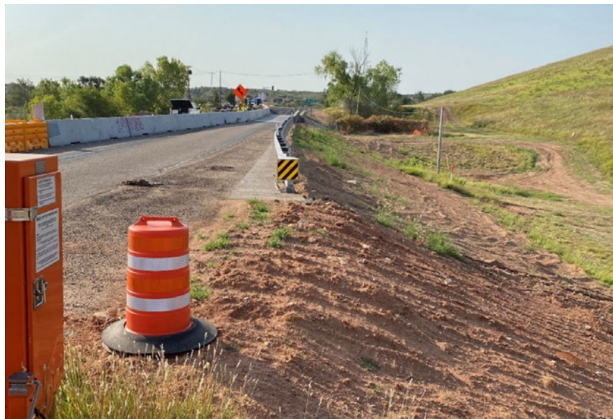
Figure 11 – Existing Bridge and Salt Fork River Crossing, Facing South
