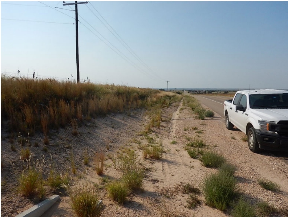
Photo 2. Typical view of SH-70 ROW in proposed Route Option A, facing south.
