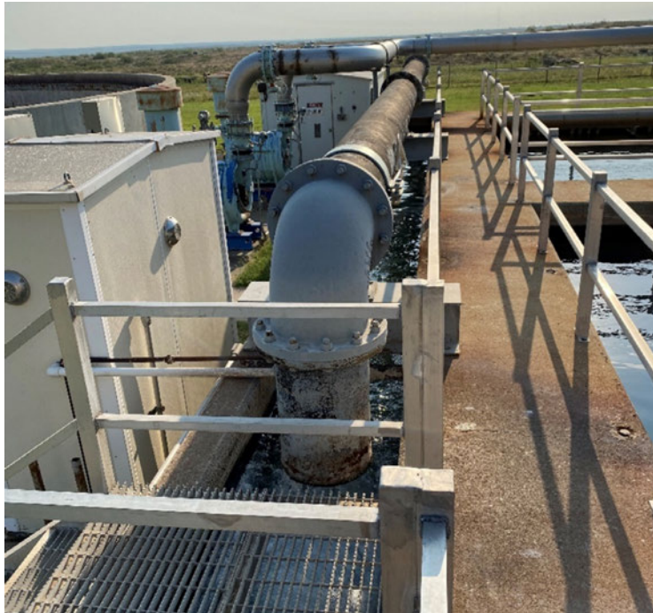
Figure 12 – Clarendon Well Field Outfall to Filters
