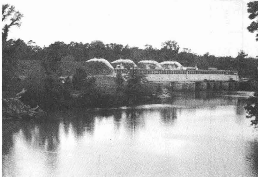
Figure 5.--Lower Neches Valley Authority Pumping Plant at Voth.
