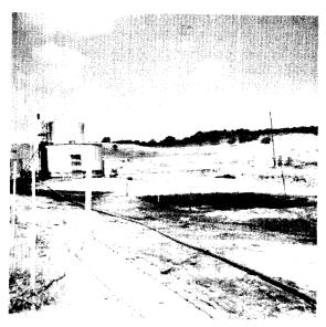
F. Tank battery location showing evidence of oil spillage and overflow. Small pit located in right center (dark area), Sec. 4, Blk. 1, ELRR Survey. View is west.
