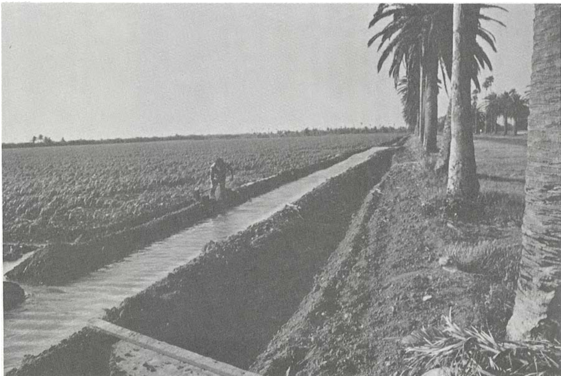
Unlined canal, used to irrigate grain sorghum with water from the Rio Grande. Much water is lost by seepage from such unlined delivery systems. Photo courtesy U.S. Soil Conservation Service.
