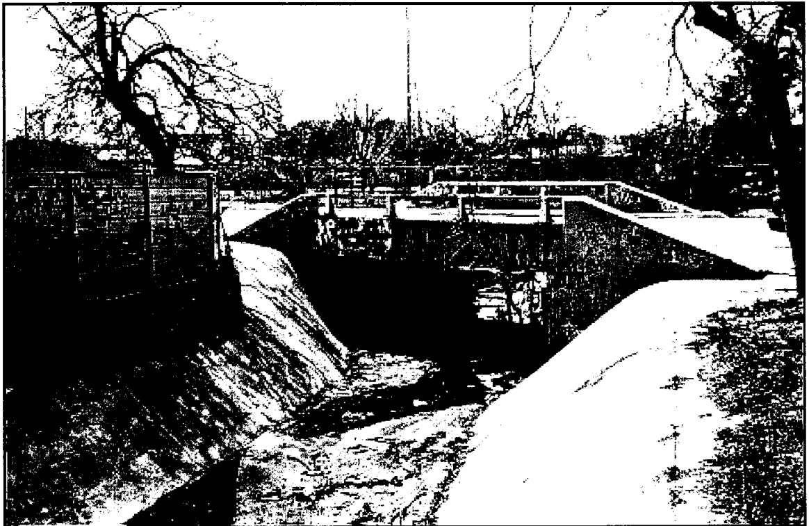
Tributary 1 Looking Downstream at Bridge at Crockett Street
