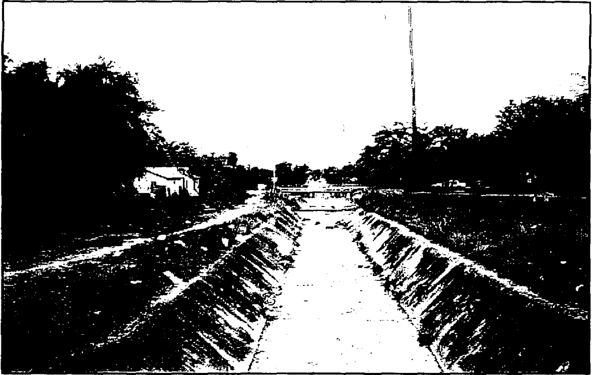
Tributary 3 Looking Downstream from Bridge at Colorado Street
