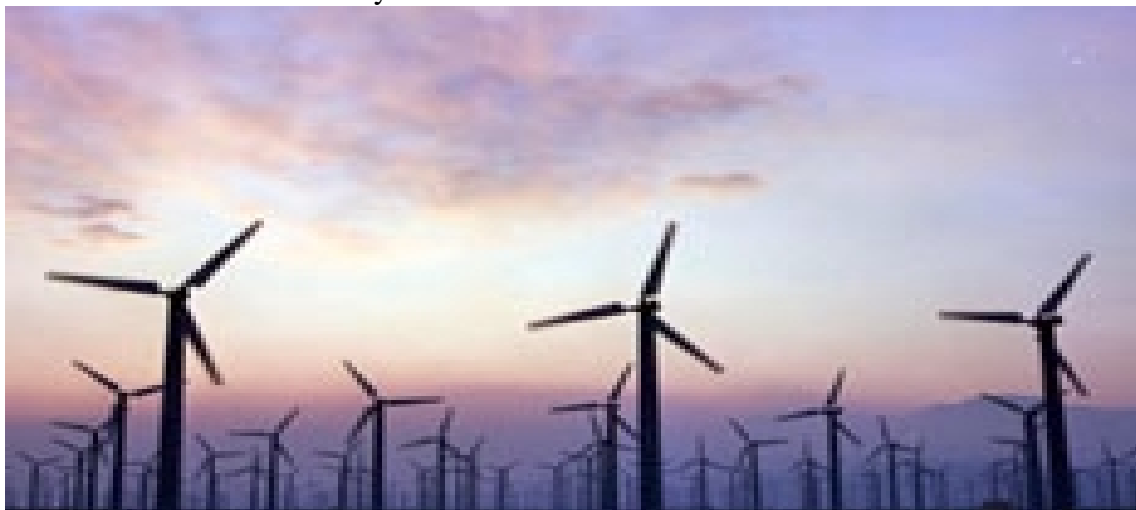
Figure 1-4 Wind Turbine Farm
