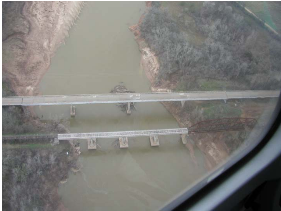
Figure 3.4 – Highway and railroad bridges at Site 1. Flow \approx 4,000cfs.
