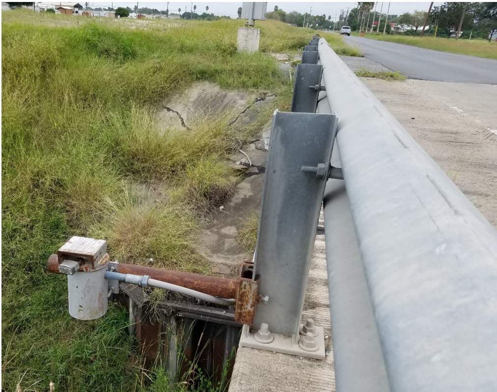
Figure 14: Typical CCDD5 Stage Gauge Setup
