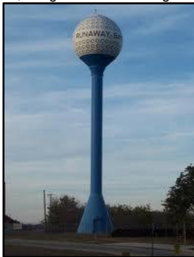
100,000 gal elevated storage tank
