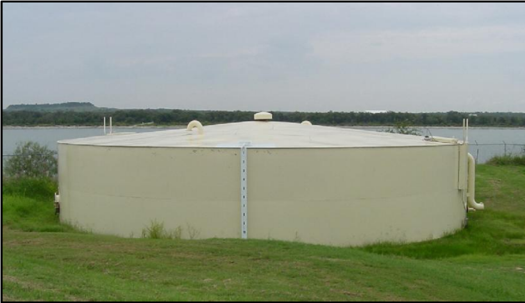
300,000 gallons storage tank
