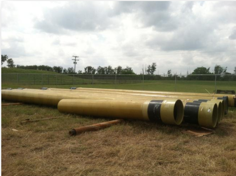
Fiberglass casing ready for installation at NAWSC
