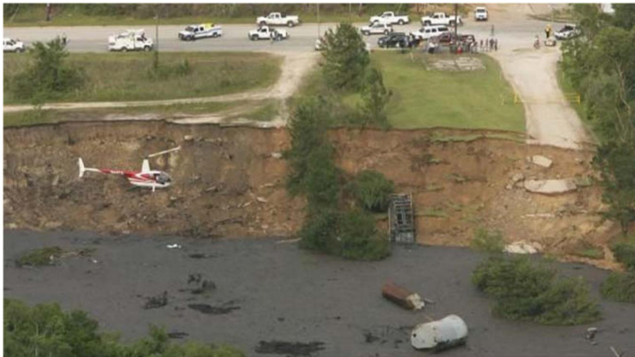
Figure 2-14 Photograph showing catastrophic collapse and sinkhole that formed over Hull salt dome in 2008 in the town of Daisetta, Liberty County, Texas (from Horswell, 2009).
