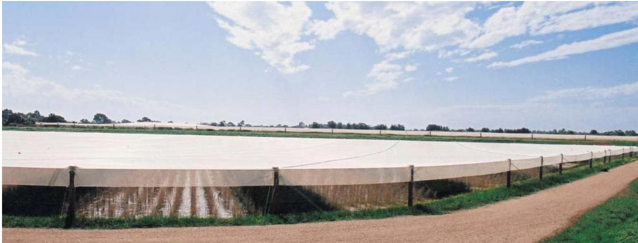
Figure 8-7: Bird-Proof Netting over the Reedbed at the Parafield Stormwater Harvesting Facility
