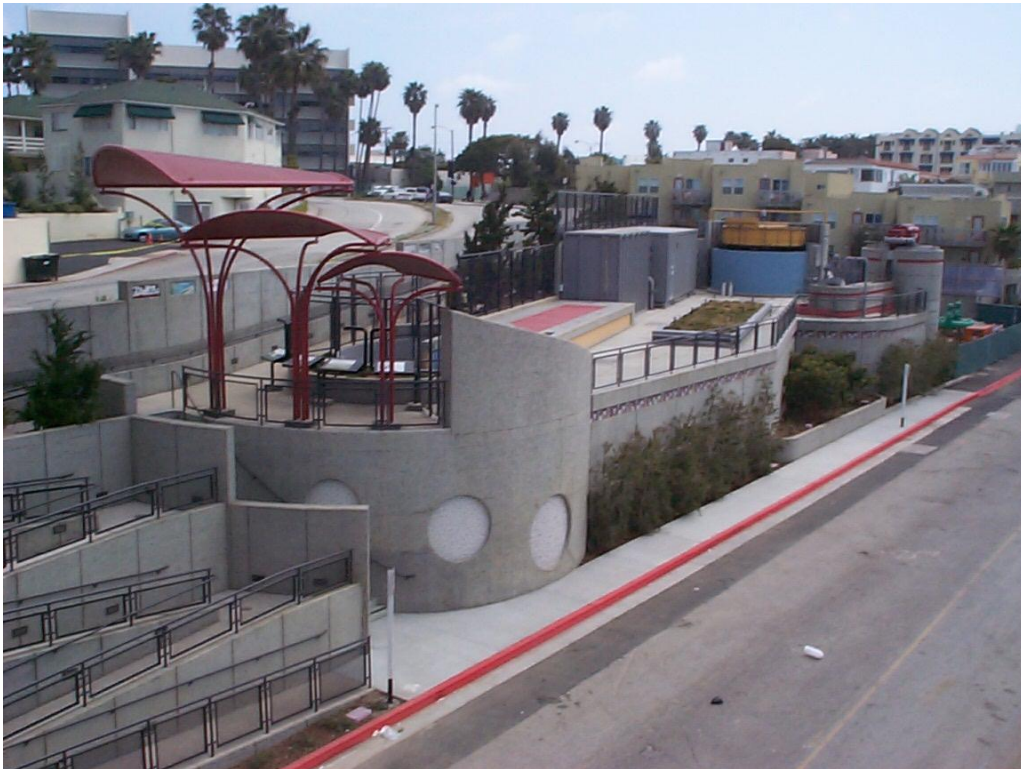
Figure 8-1: Santa Monica Urban Runoff Recycling Facility
