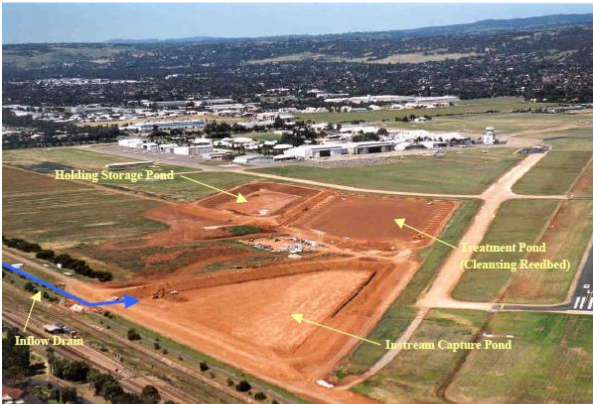
Figure 8-6: Construction of the Parafield Stormwater Harvesting Facility
