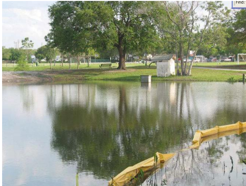
Figure 8-5: Detention Pond at the Winter Park Civic Center
