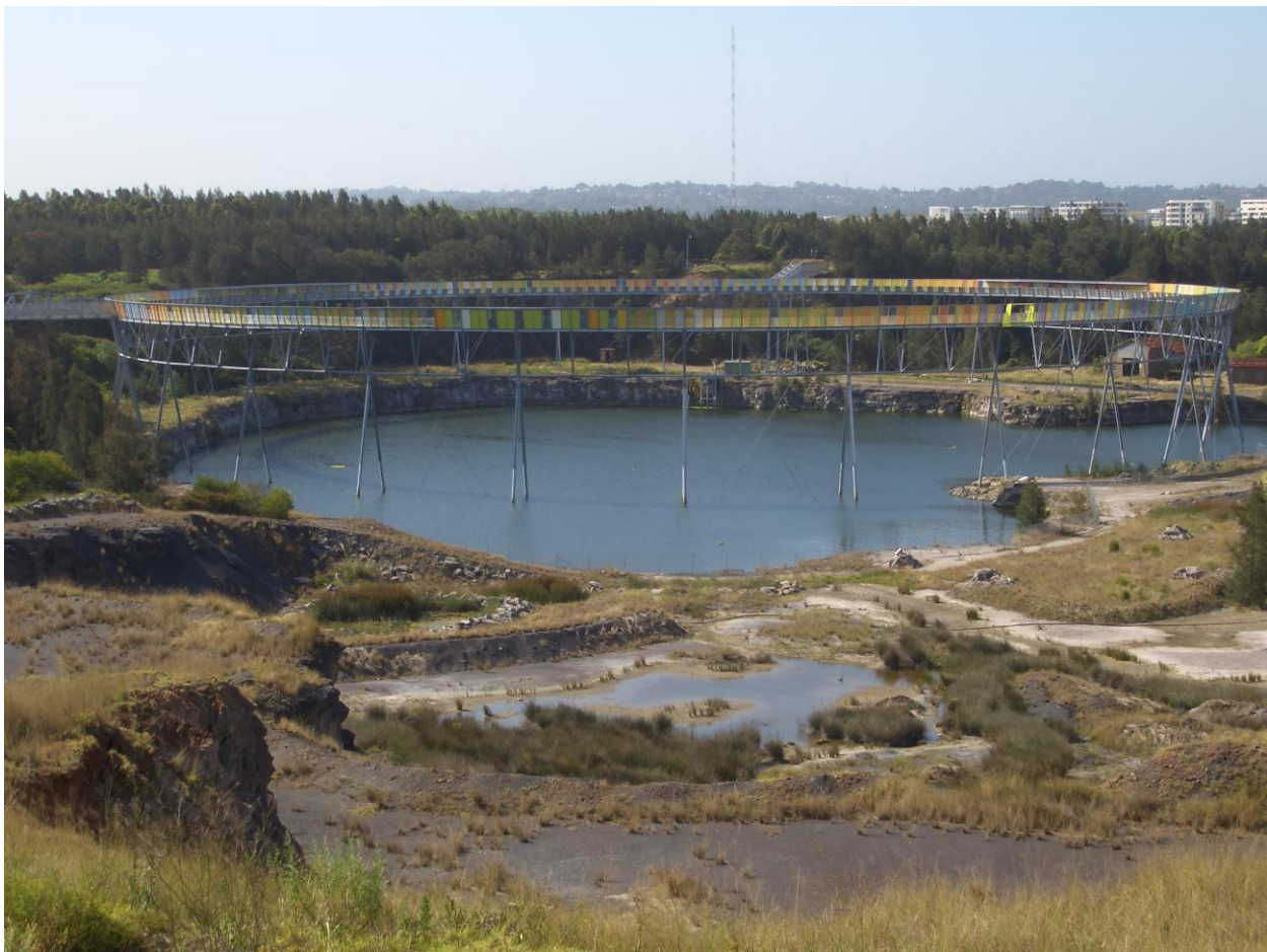
Figure 8-8: Brick Pit Storage at Homebush Bay
