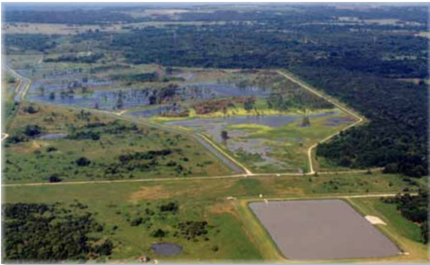
Tarrant Regional Water District uses constructed wetlands to further “polish” wastewater-dominated river water withdrawn from the Trinity River as a method of indirect reuse.
