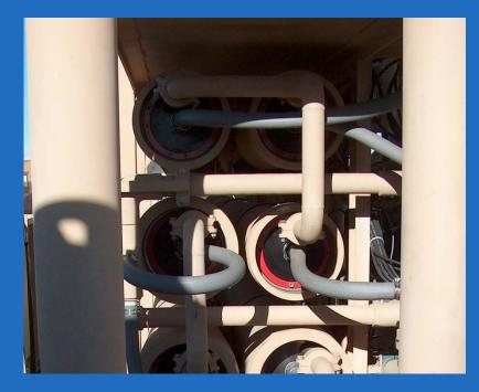
Use the Second Pass Manifold to connect vessels 1 and 4 to 5.
