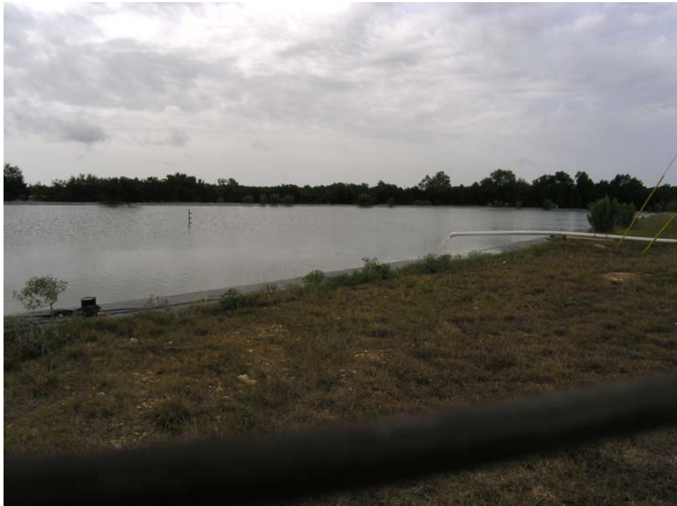
Figure 12-7. View of River Oaks Ranch evaporation pond showing concentrate outfall and water-level gage
