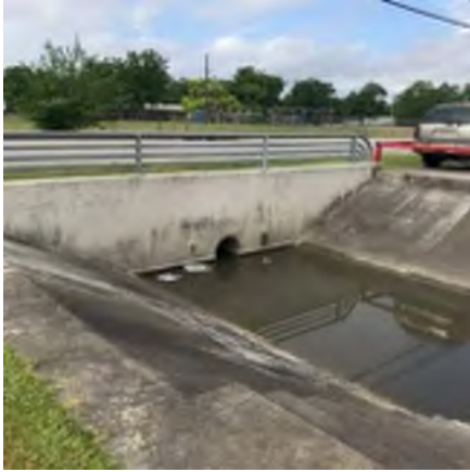
Figure 2-1: 24-inch culvert outfalling into the upstream end of P118-27-00
