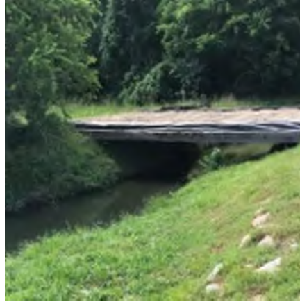
Figure 2-2: Temporary Pipeline Easement Wood Bridge
