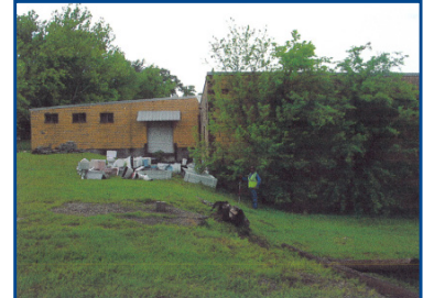
Picture 3. Back Side of Building Facing South 3/28/2012
