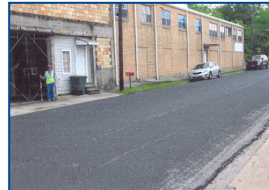
Picture 6. Left Side of Building 3/28/2012
