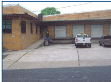
Picture 2. Front Side of Building Facing North 3/28/2012
