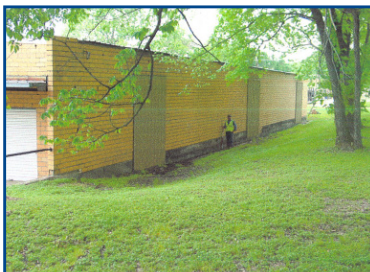
Picture 4. Right Side of Building 3/28/2012
