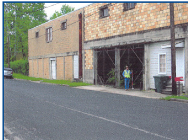
Picture 5. Left Side of Building 3/28/2012
